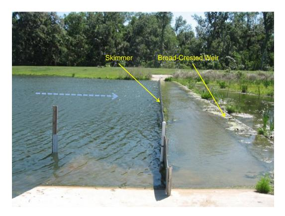
Figure 1-5. Broad-crested Weir Structure.
